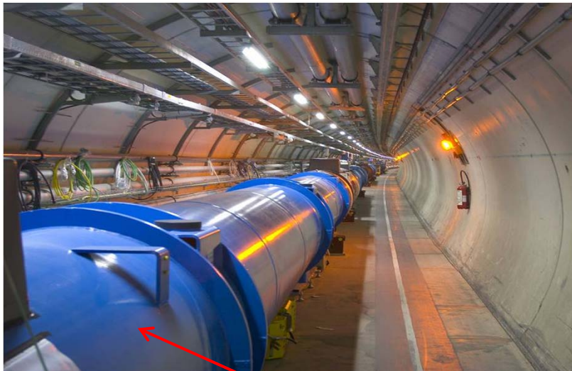
superconducting magnets (inside acryostat)
